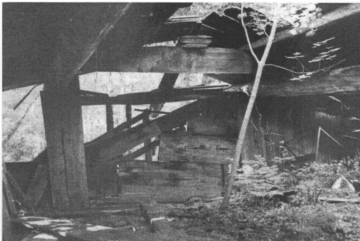
Figure 16:2. Interior of Planked Post-and-Beam House, FeSr 1, 1970. (Photo: P.M. Hobler).
