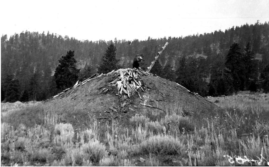
FIGURE 3.7B. *A photograph of one of the few remaining pithouses at the turn of the century. Note in particular the earth covering and notched log ladder.*
