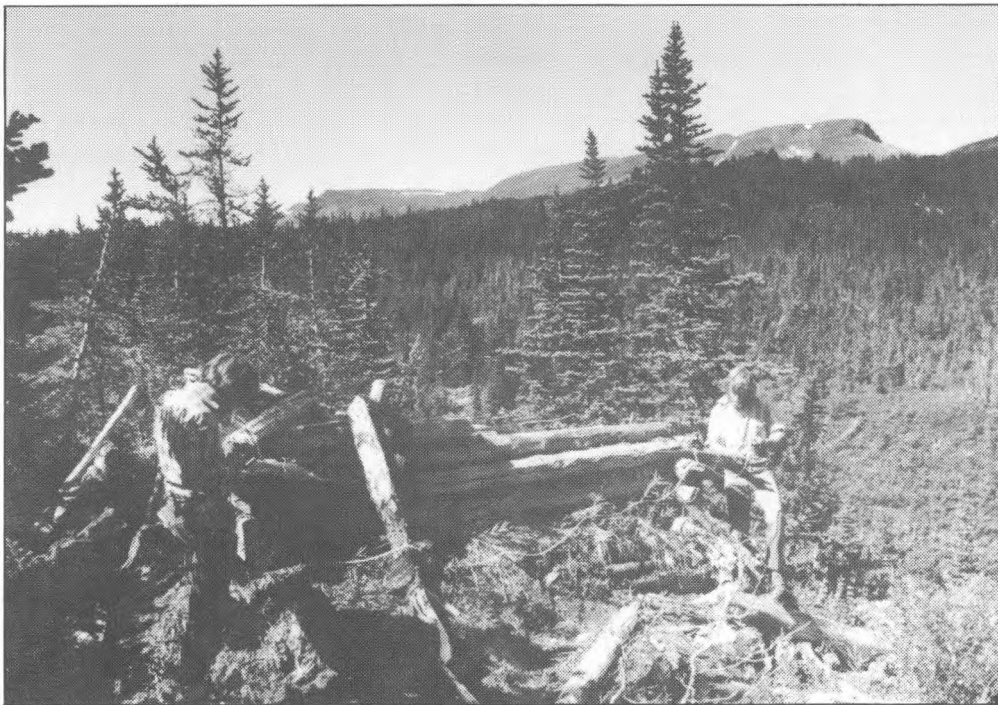
Fig. 42. Bourgeaux Creek telegraph line-cabin (EH-1), Bourgeaux Valley. View of east wall looking northwest.
